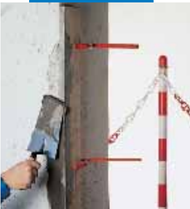
Repairing vertical arrise with Nivorapid
