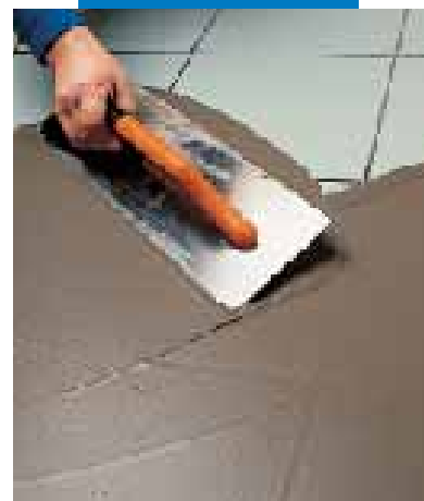
Levelling of existing floor with Nivorapid
