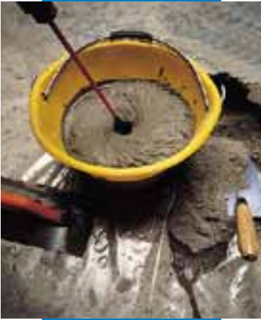
Nivorapid mixed with mechanical mixer
