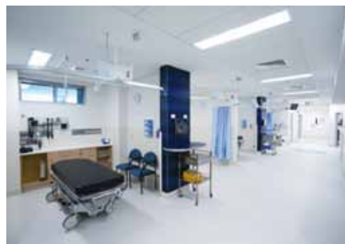
Geelong Hospital - Vinyl installed at the Geelong Hospital Emergency Department after the concrete was levelled with Ultraplan
