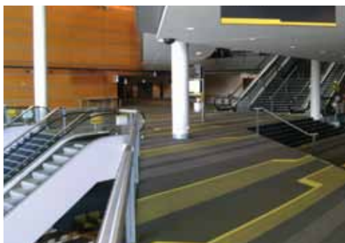
Brisbane Convention Centre - Carpet installed at the Brisbane Convention Centre after the concrete was levelled with Ultraplan
